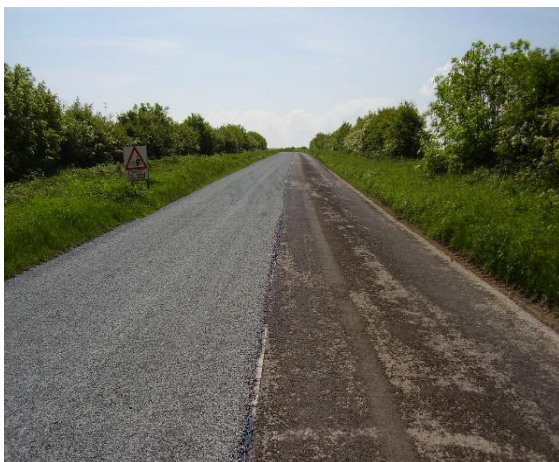
Image Two – New surface & Old surface
