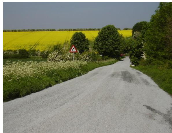
Image Three – Completed surface
